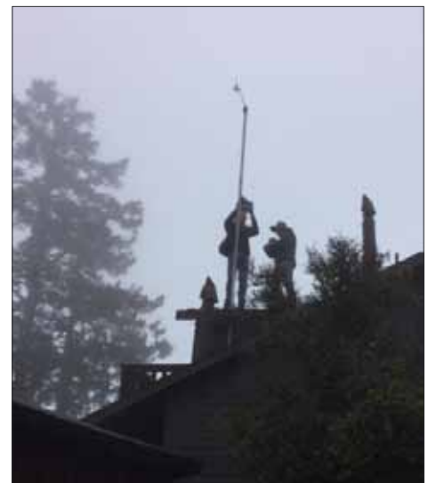
Innkeeper Gordon Edwards and CAC Member Tim Aaronson installing the weather station on the roof of West Point Inn.
